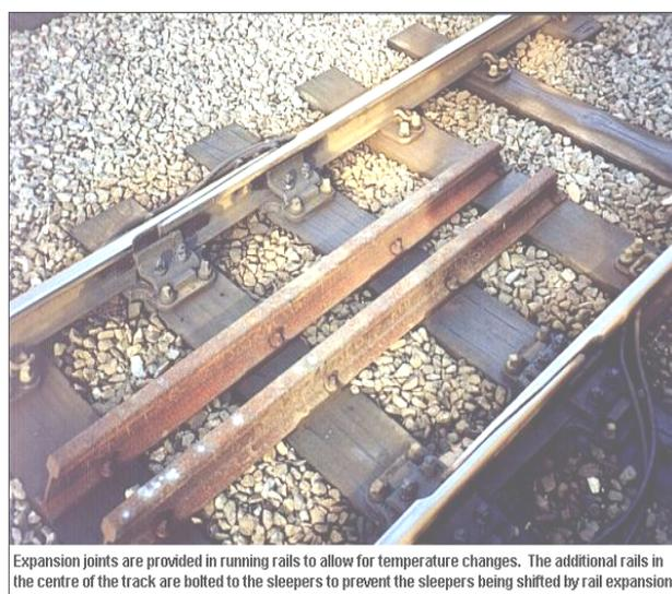
Expansion joints are provided in running rails to allow for temperature changes. The additional rails in the centre of the track are bolted to the sleepers to prevent the sleepers being shifted by rail expansion.
